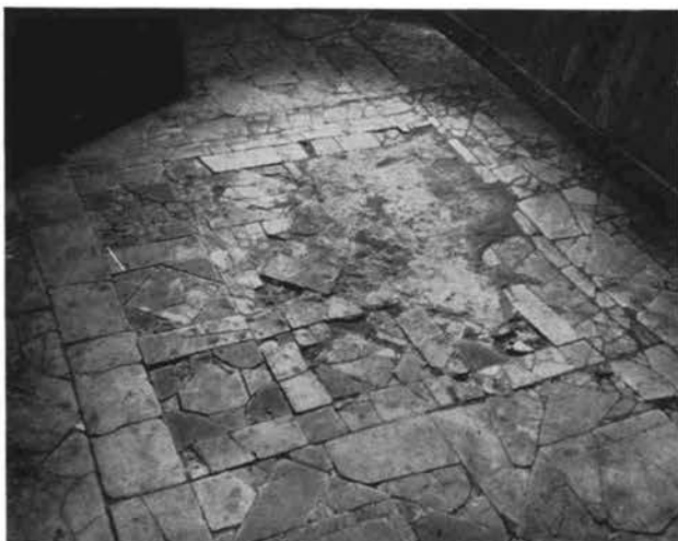
Fig. 187 — S. Marco. Panel in sectile pavement (Photo: Corbett).
